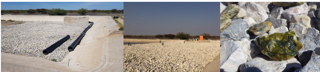
Figure 3: Rock filter under construction (with visible collection pipes), the finished filter and biofilm (Photos: EPoNa joint project)
