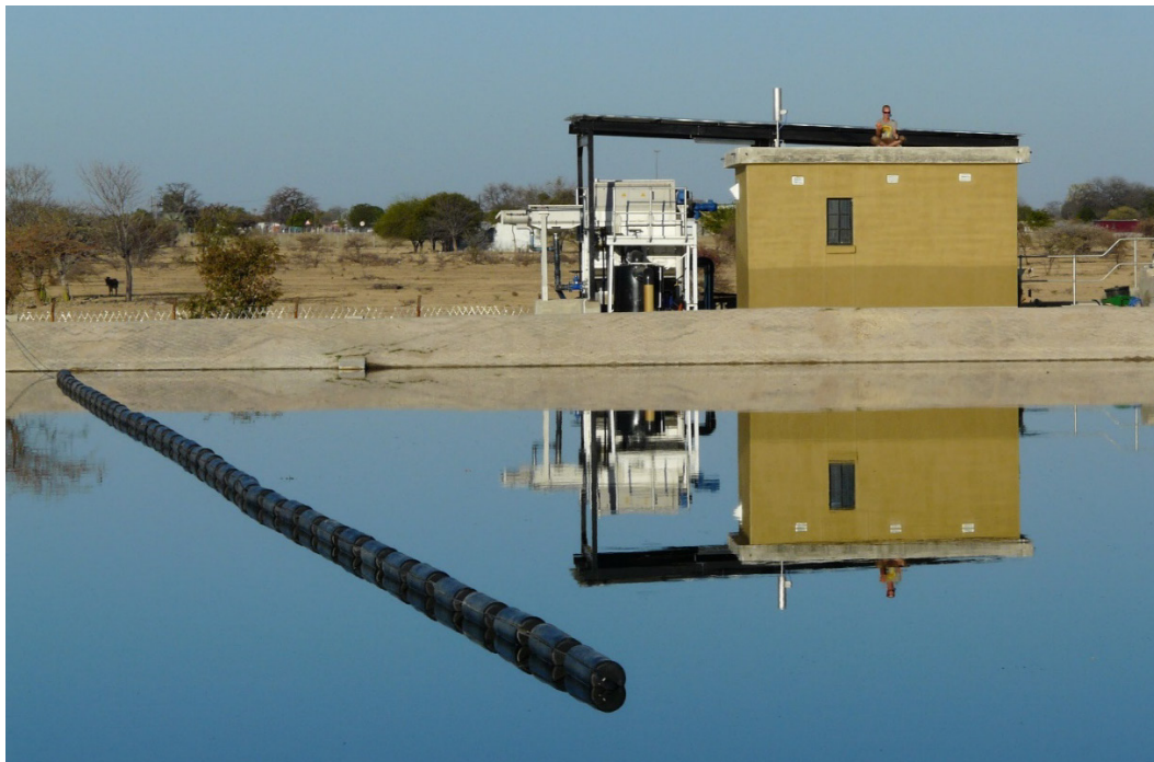
Figure 2: Pond A-1 and the pre-treatment plant (Photo: EPoNa joint project)
